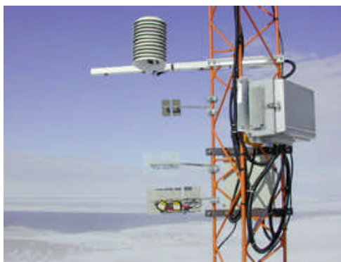
Specimens and instruments affixed to tower at exposure site
