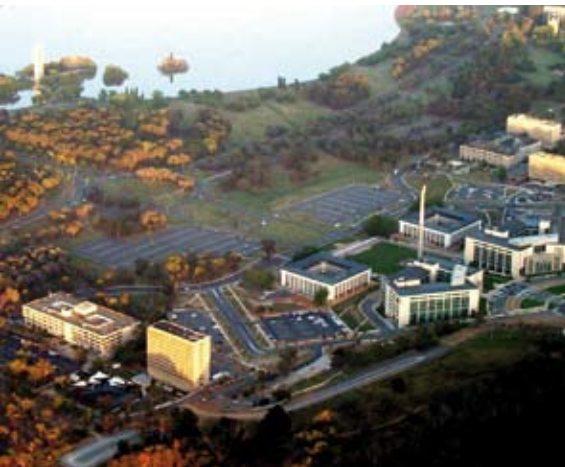
The Russell Offices in Canberra which house, along with the Department of Defence, ONA, ASIO, DSD, DIO and DIGO.
