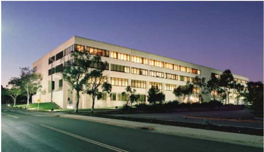
The ASIO-ONA Building
