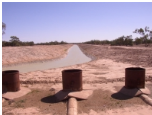
Figure 3: Excavated channel from Lake Cawndilla to the Darling River
